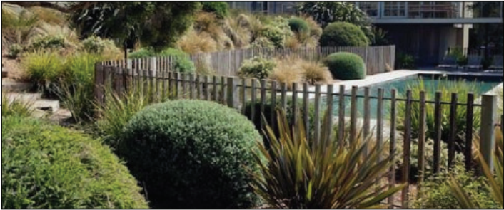
Regulation pool fencing concealed by shrubs and plantings with 900mm clearance from pool barrier
