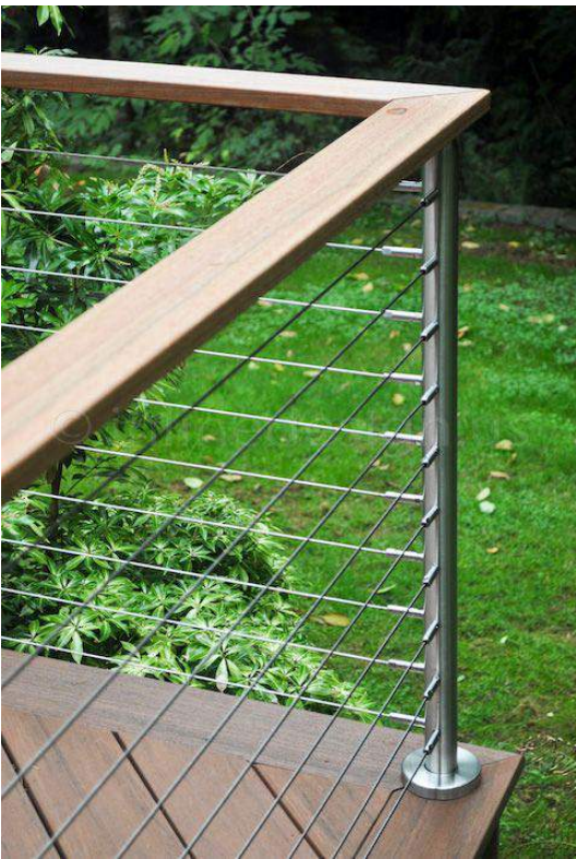
WIRE BALUSTRADE WITH TIMBER HANDRAIL
