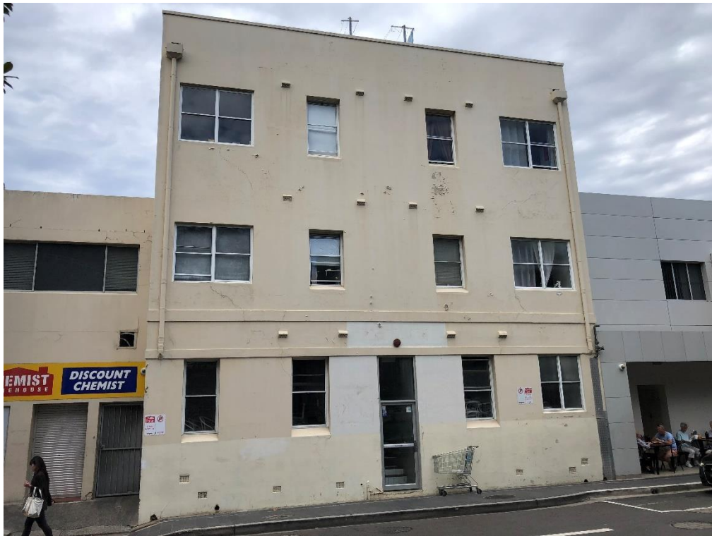
Figure 21 - North (rear) elevation of 19-21 The Corso, Manly.
