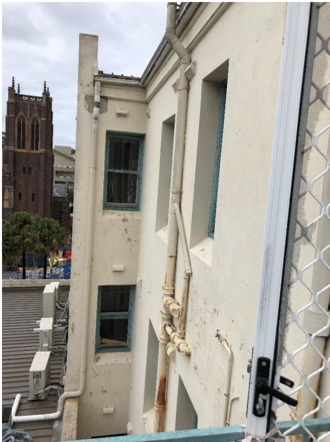
Figure 25: View across lightwell on north-east side of the building.
