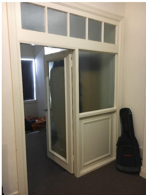
Figure 28: Second floor north unit with early but modified door detailing of the former porch entry.
