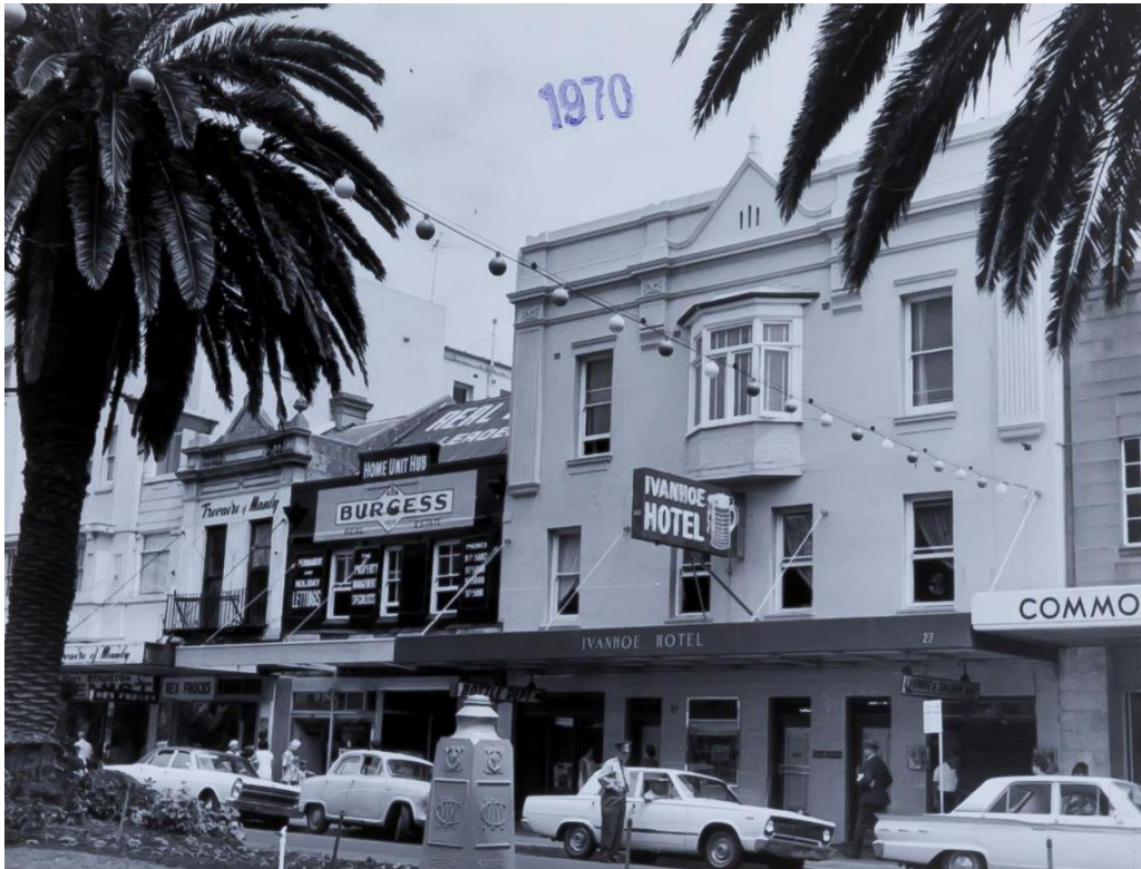
Figure 13 – 1970 photograph of the Corso, with 'Exeter Flats' on the far left and Trevaire's still located at 23 The Corso. (Source: Australian National University, Noel Butlin Archives Centre, Tooth's Yellow Cards, 'Plaza Hotel (ex Ivanhoe Hotel to 1978), The Corso, Manly', Card 7 Side 2, N60-YC-533)
