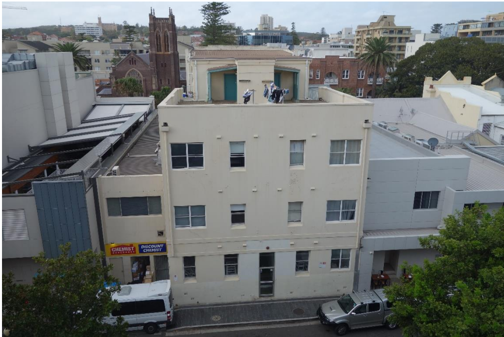
Figure 33 - View from top floor of carpark looking over 19-21 The Corso to the south.
