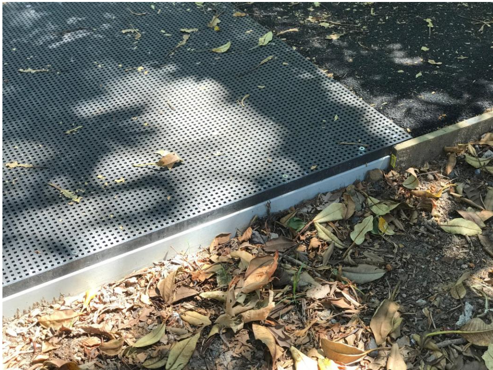
Plate 2 – Typical elevated FRP walkway interface with asphalt path (St. Leonards Park, North Sydney)
