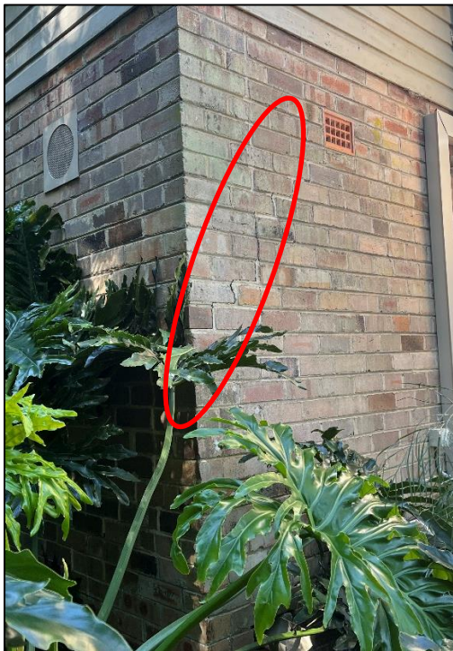
Photographs 4 and 5: Cracking within the rear of the site residence.
