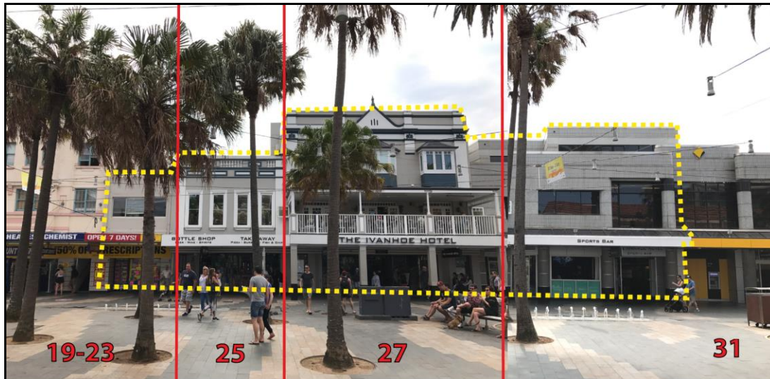
Figure 1: Indication of Subject Site (Images by Alexander & Co)
