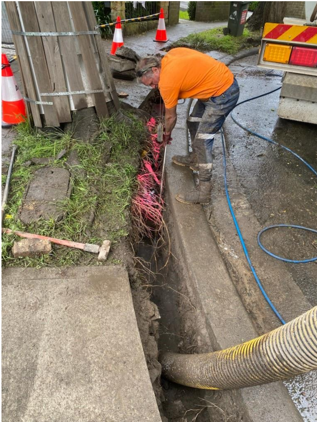
A Vac truck is used to expose roots so services can be placed underneath tree roots.
