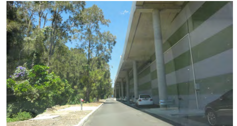
The interface between No. 6 Jacksons Road and the multi-level car park
