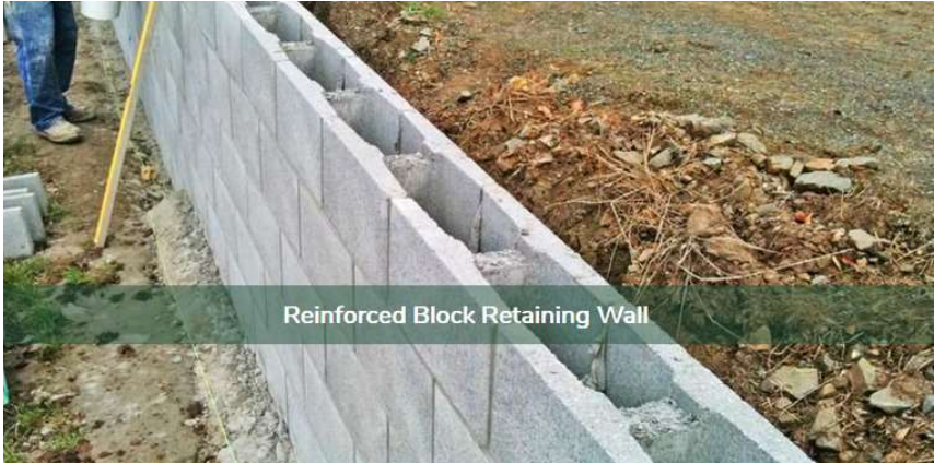
REINFORCED BLOCK RETAINING
