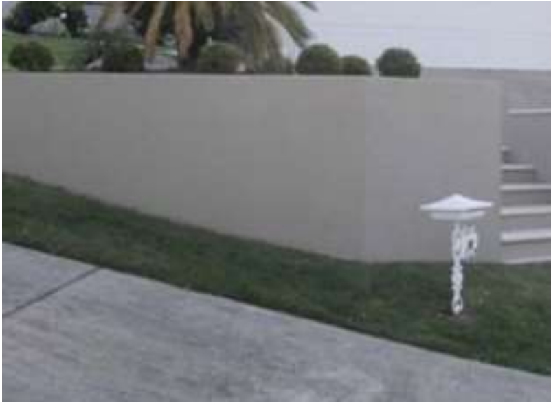
RENDERED STRUCTURAL BLOCK WALL
