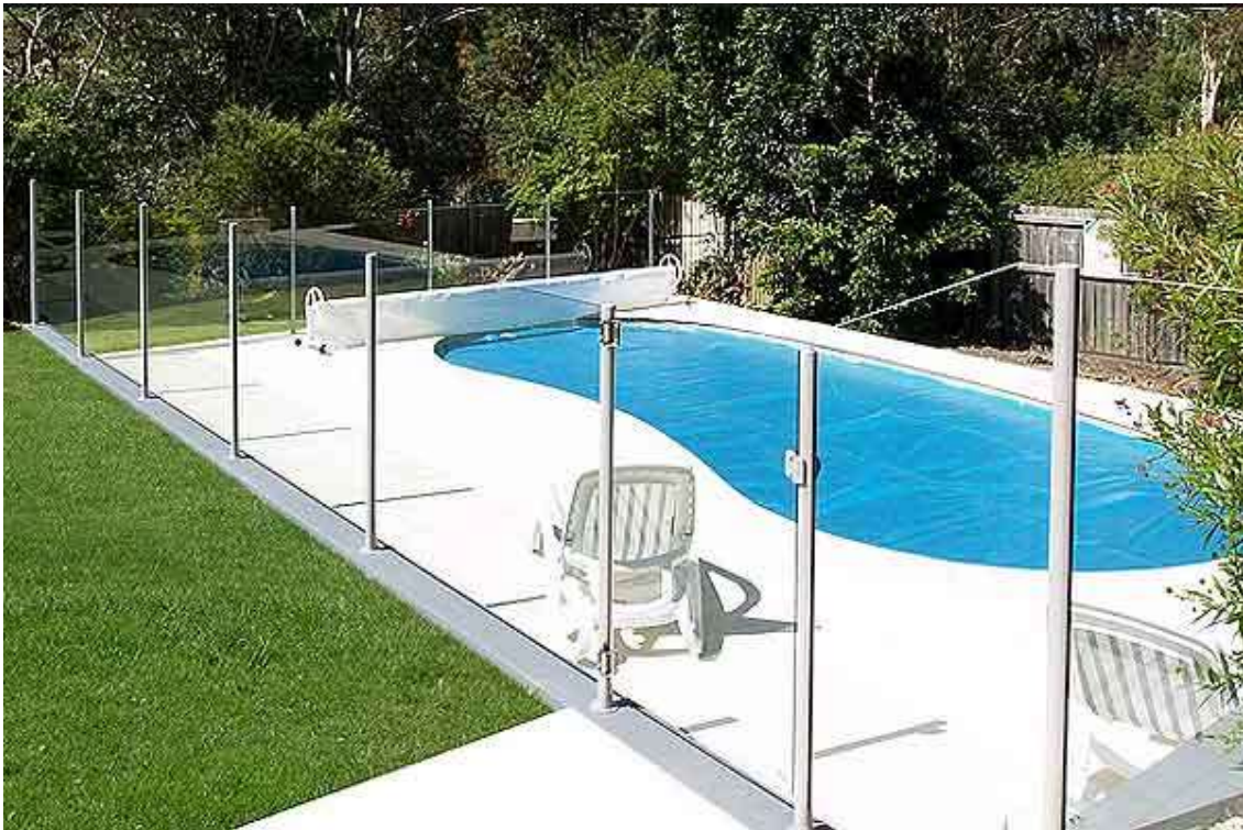
SWIMMING POOL FENCING—TO COMPLY WITH POOL FENCING ACT
