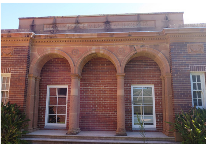
Remnant façade of Building 1
