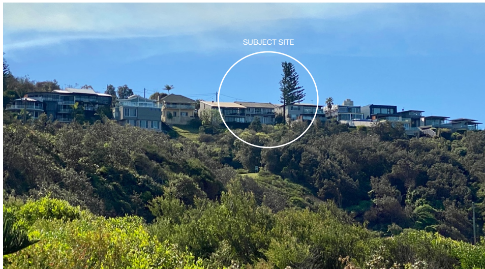
Subject site (behind Norfolk Island Pine at centre) as seen from Newport Beach.
