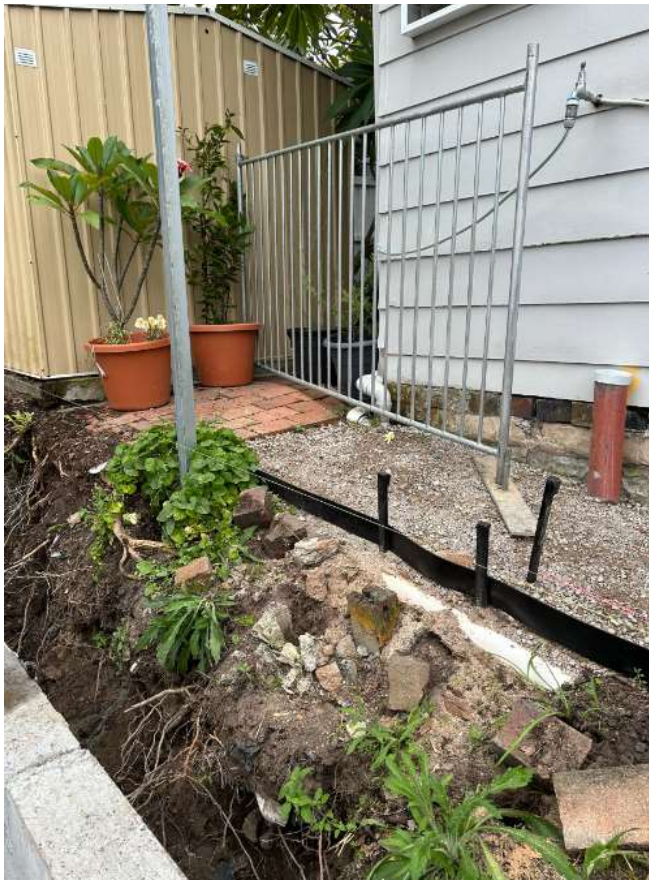
Photo 1: Location of stormwater pipe
