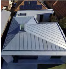
METAL ROOF SHEETING -STANDING SEAM
