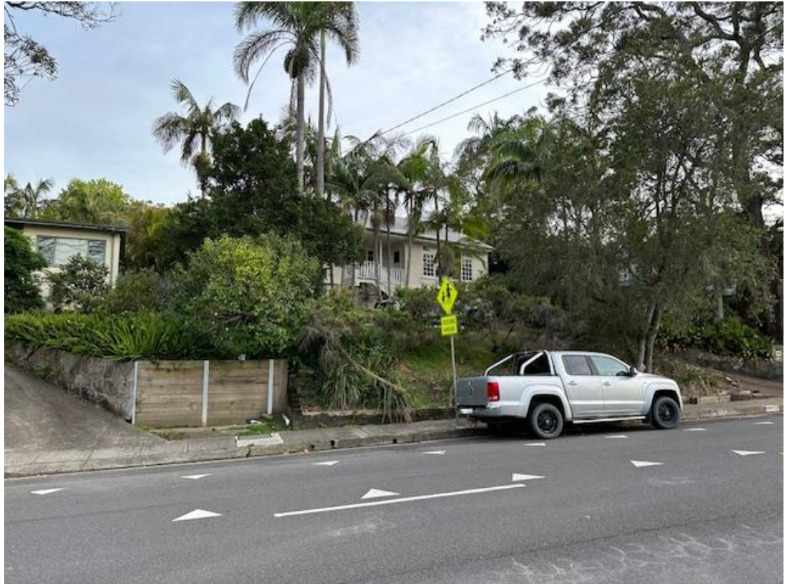
Figure 6 - Photograph of adjoining dwelling house to the east 52 Beaconsfield Street
