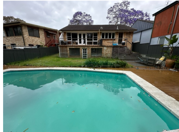
Photo 2: Rear of the dwelling facing south.
