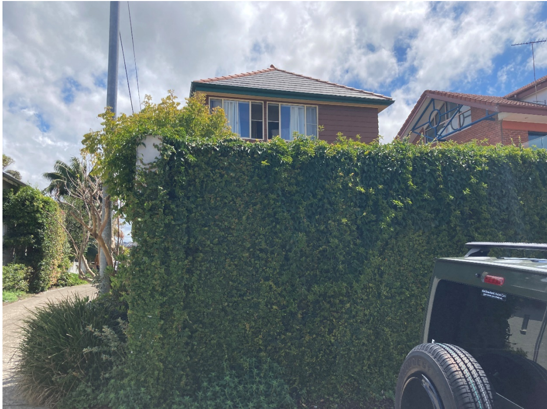
Photograph 2: Upper-level window, 18 Addison Road.
