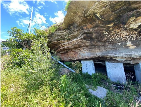
Outcrop cliff and underpinning at north-west corner of No. 2
