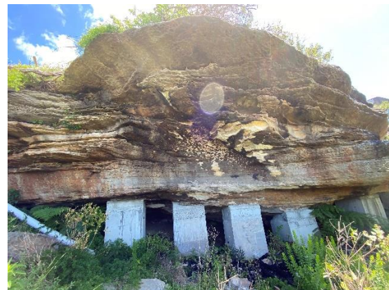
Outcrop cliff and underpinning at north-west corner of No. 2
