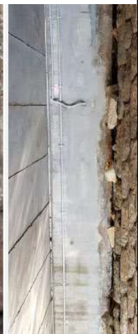
Photo No: 27 Ab Evidence of possible settlement
