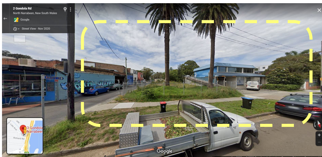
Photo 2 – View of subject site looking north along Gondola Rd – 1-3 Gondola Rd in the foreground
