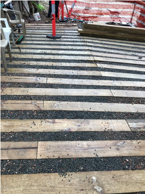
Figure 7 Sleepers with gravel between protecting ground from compaction
