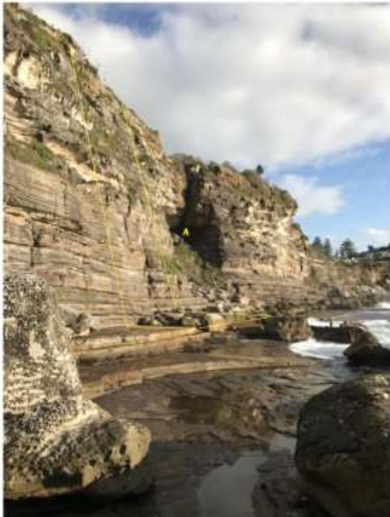
Figure 4: View of cliff face and rock platform at subject property on 7 April 2018, looking NW, with approximate lot boundary depicted, and St Michael's Cove visible in background at "A"
