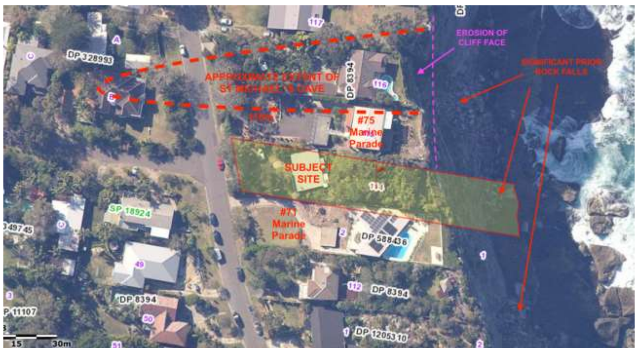
NSW Gov Six Maps extract marked up to show: Significant Rock Falls to the rock platform from the subject site. Erosion of Cliff Edge to St Michael's Cave. Extent of 110m Cave under adjoining properties, roadway, footpath zones and Council land.
