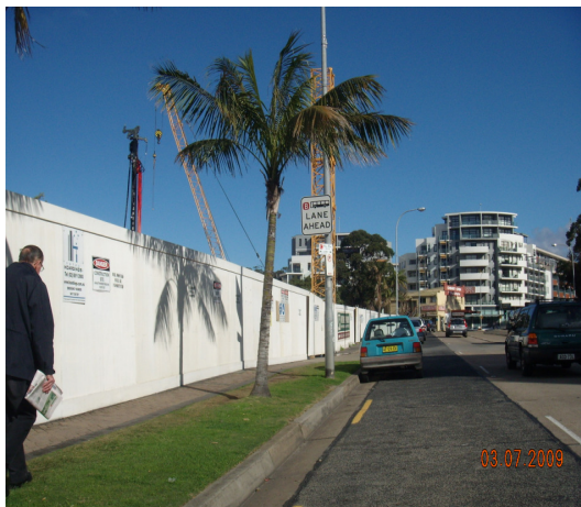
Photo 1: Pittwater Road Frontage
