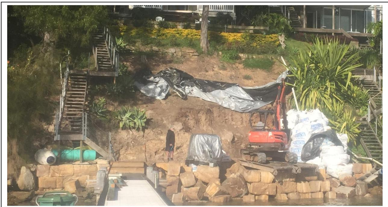
At the back of the removed sandstone block wall a cut face with a height of about 2.5m had been created. The materials exposed in this cut comprised approximately 1.6m of clay fill overlying natural clay and extremely weathered siltstone bedrock. Siltstone bedrock of at least very low strength was exposed at the
