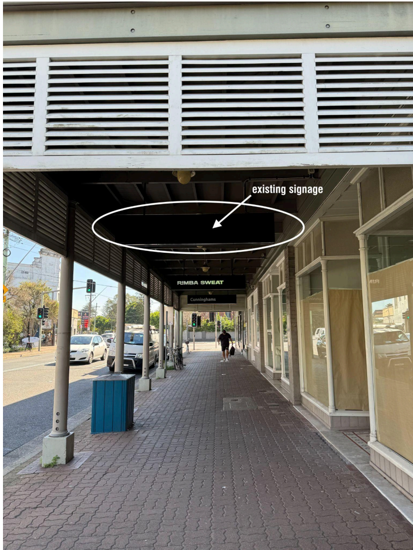
Figure 1. Photo along arcade showing subject shop's (on the right) existing signage.
