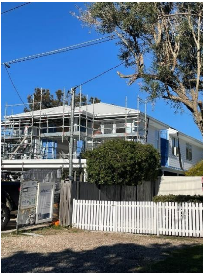
9 Lido Ave. currently under construction June 2024
