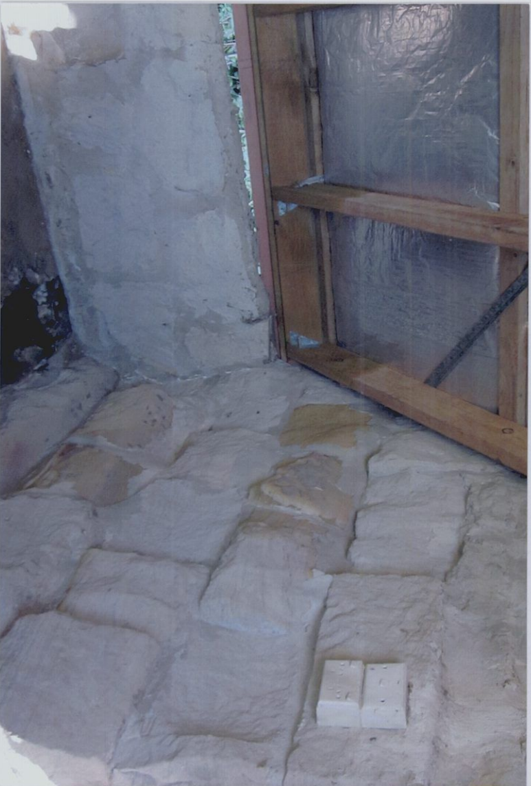
Rough interior wall of ensuite west & south walls
