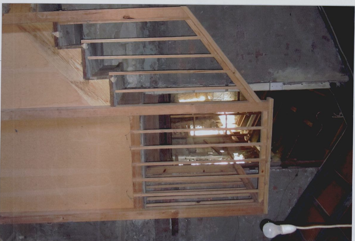
Pine staircase (not original) leading to dungeon room
