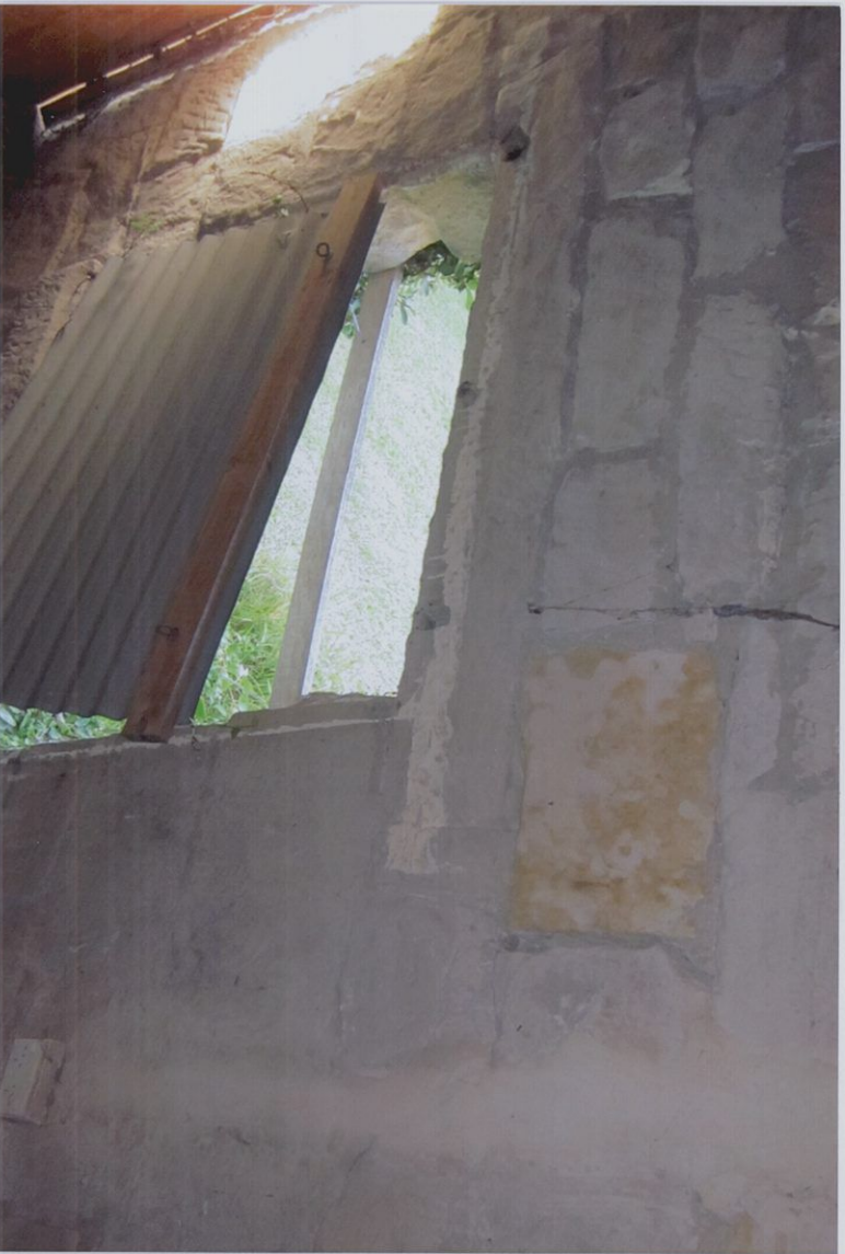
Detail showing window on east side of dungeon room. This was originally a sliding window but afforded little protection from drafts against the rough stonework.
