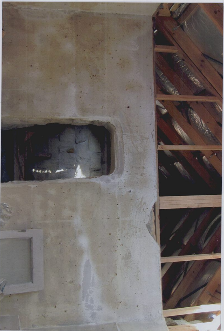
Looking from living area towards main bedroom. Note walls in this room are stuccoed/rendered to look like stone blocks.
