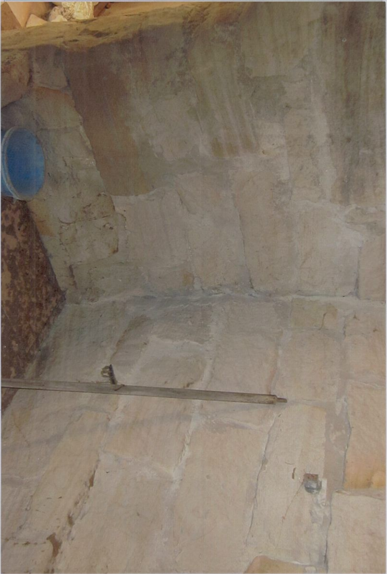
Detail of rough coursed wall in main bedroom Floor is timber.
