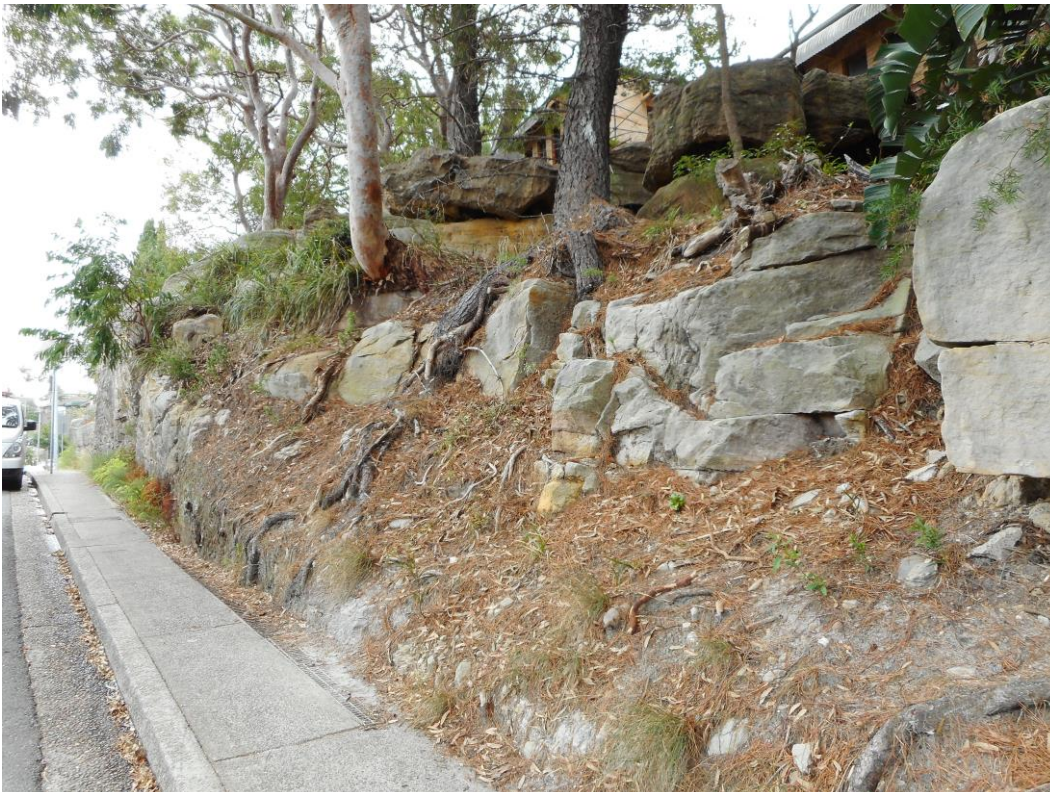
Figure 4 Existing rockface along St David Avenue boundary Source: Mecone
