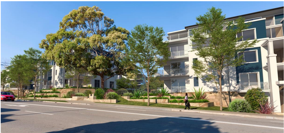
Figure 18 View from the west on Fisher Road Source: Rose Architectural Design
