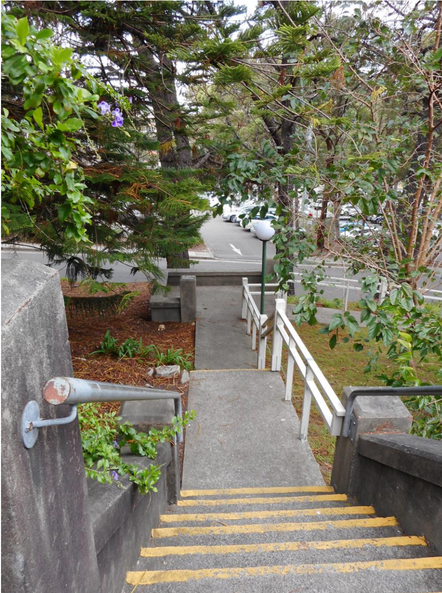
Figure 5 Existing stair access to Pacific Lodge looking towards Civic Drive to the east Source: Mecone
