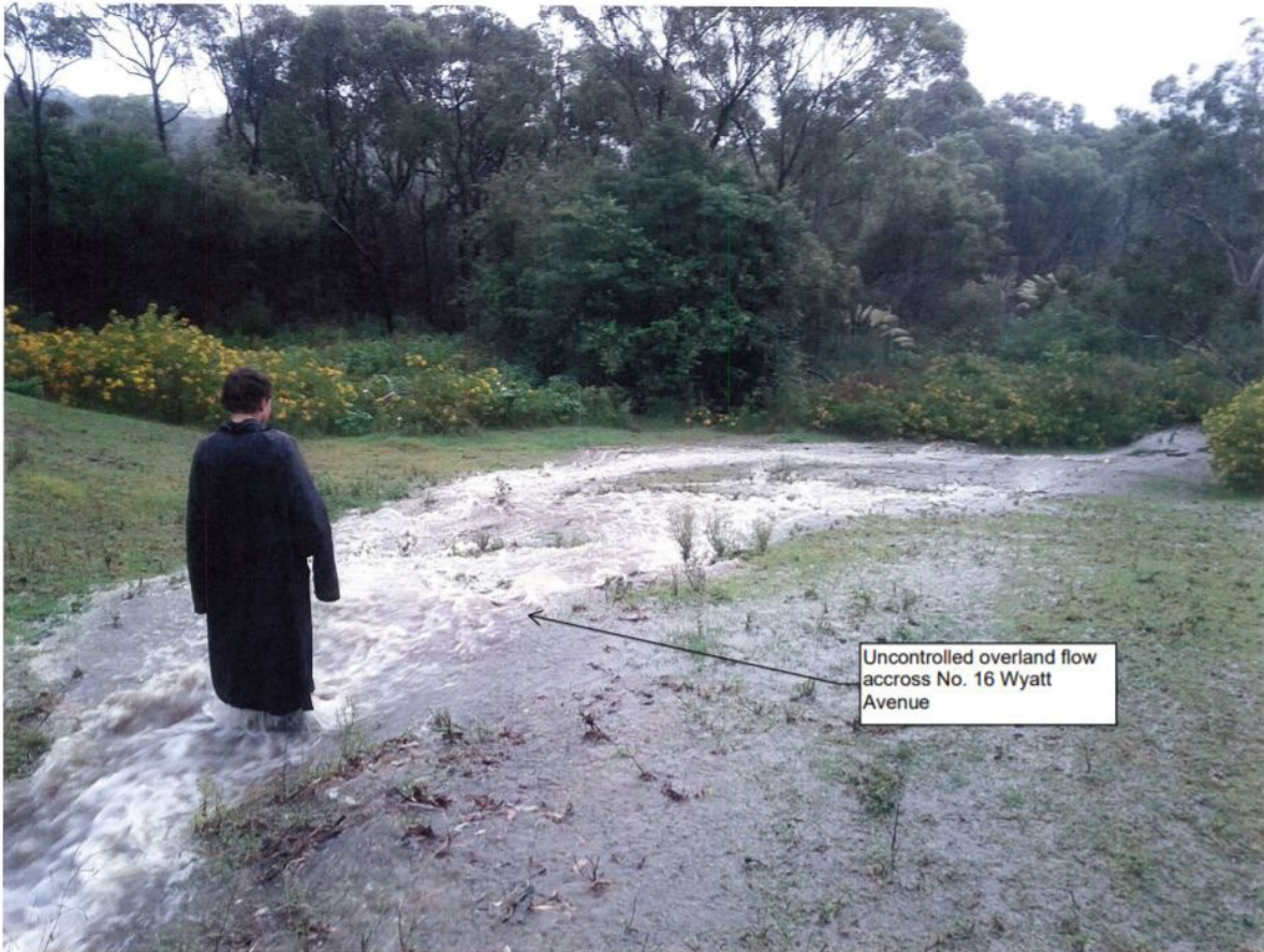
Photo 2. Stormwater flooding at the rear of No 16 Wyatt Ave looking North towards the bushland in the adjoining Property at the rear of No 16 Wyatt Ave.
