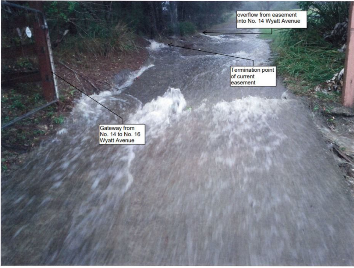
Photo 1. Stormwater flood at the rear boundary of No 14 Wyatt Ave looking north into the rear of No 16 Wyatt Ave
