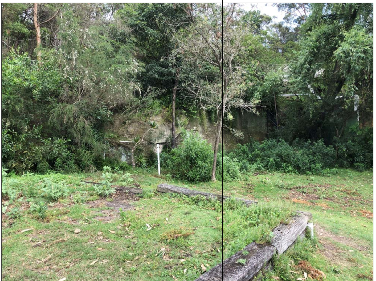
4 ROCK OUTCROP ACROSS SITE
