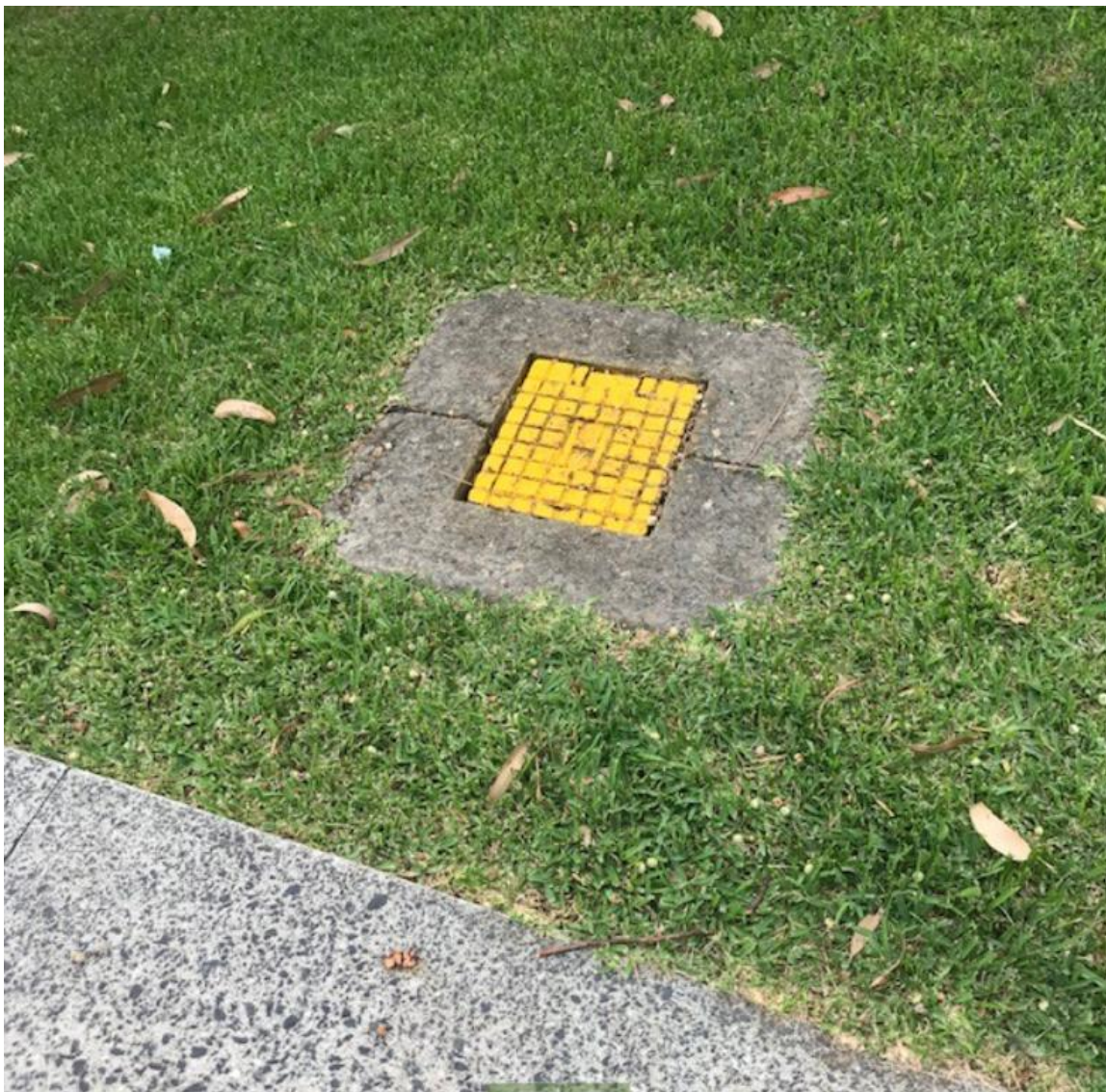
Photo 10 – Indicates the reticulated mains pressure fire hydrant located outside No.29 Ralston Rd (Steve Brooks 2025)
