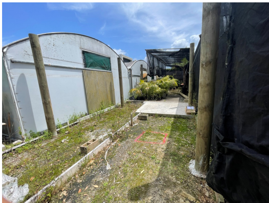
Photograph 6: Fibro-cement wall material on the glasshouse.
