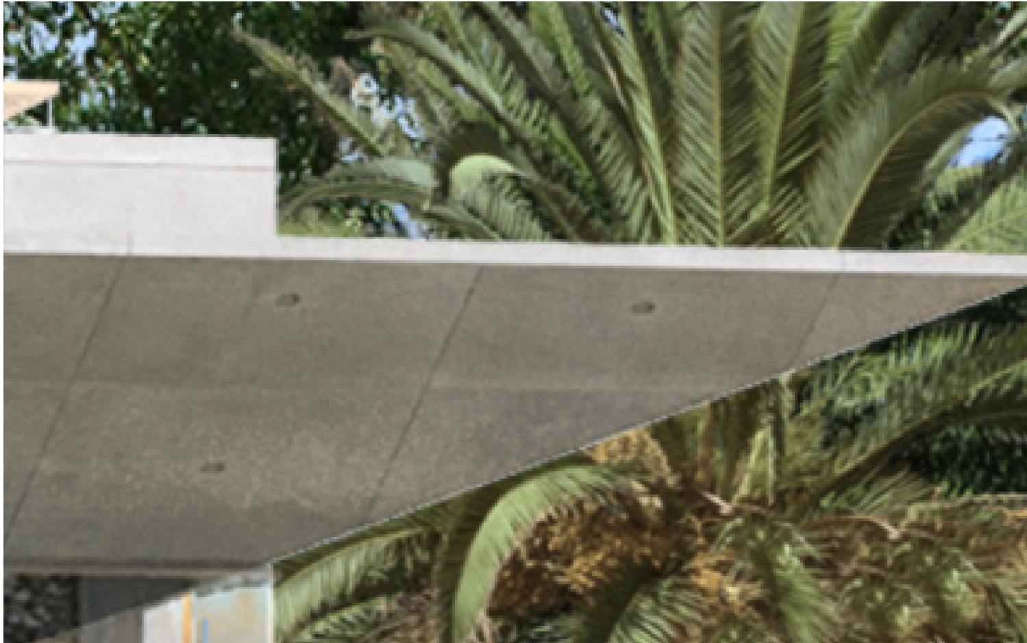
off form concrete to roof and roof soffits
