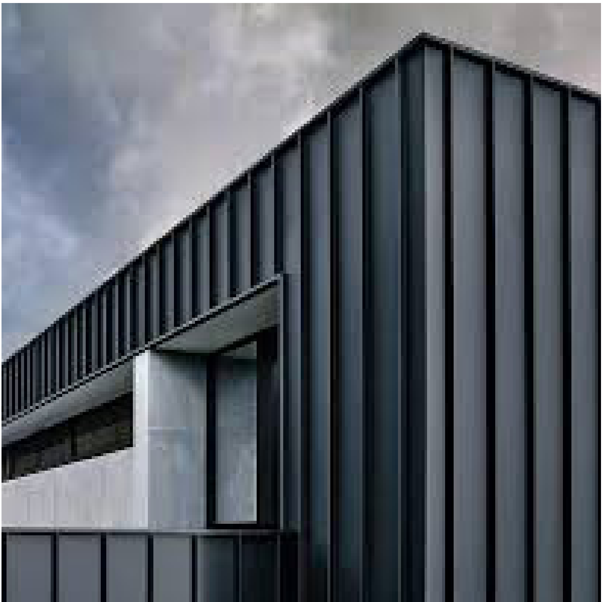
metal cladding - black - to lower walls (for thermal performance)
