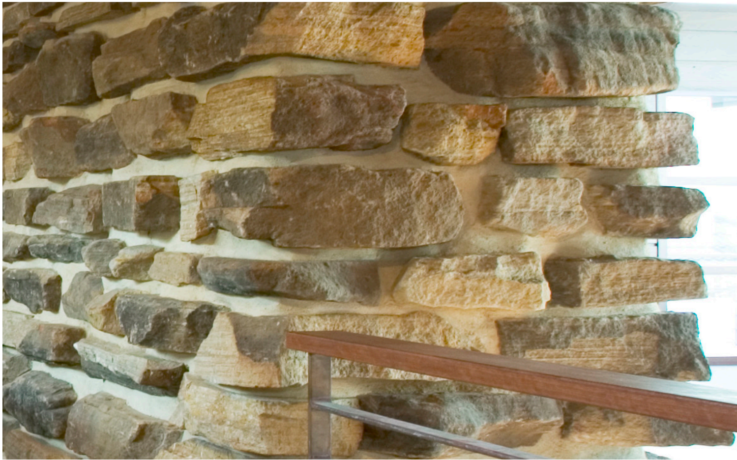
sandstone rubble walls to basement walls + landscape walls
