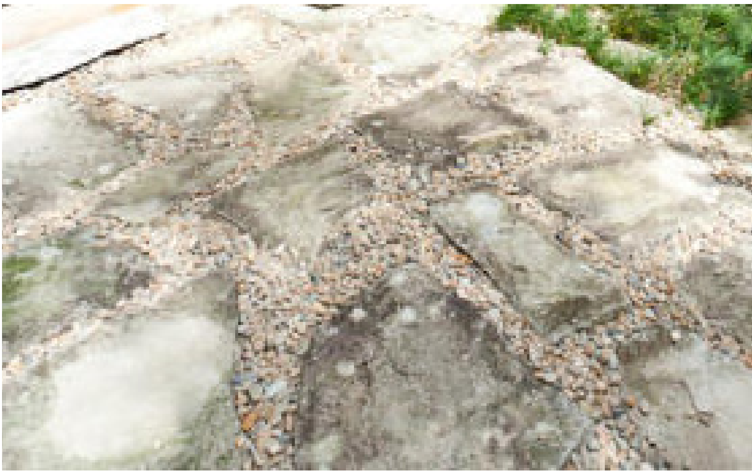
re-cycled sandstone paving to external land- scape areas and terraces - Note: Pebble to gaps
