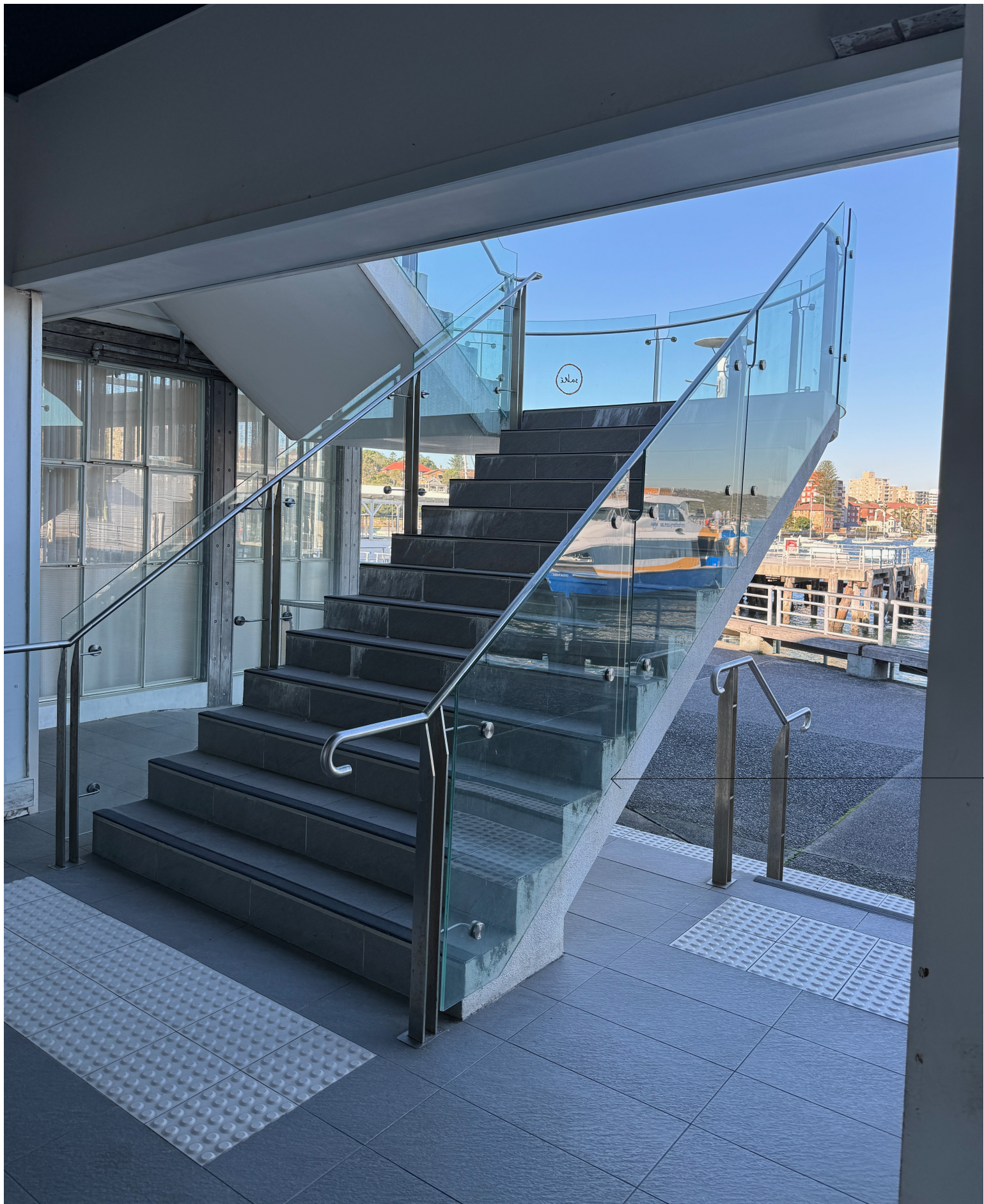
NEW STAIR AT PUB + MICRO BREWERY ENTRY CONCRETE STAIR RENDERED AND PAINTED WHITE AND FRAMLESS GLASS BALUSTRADE TO MATCH EXISTING
