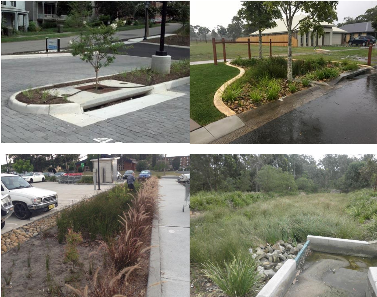
Figure 7-7 Biofiltration measures (top left clockwise) - Tree pit filter, stormwater garden, biofiltration basin, biofiltration swale
