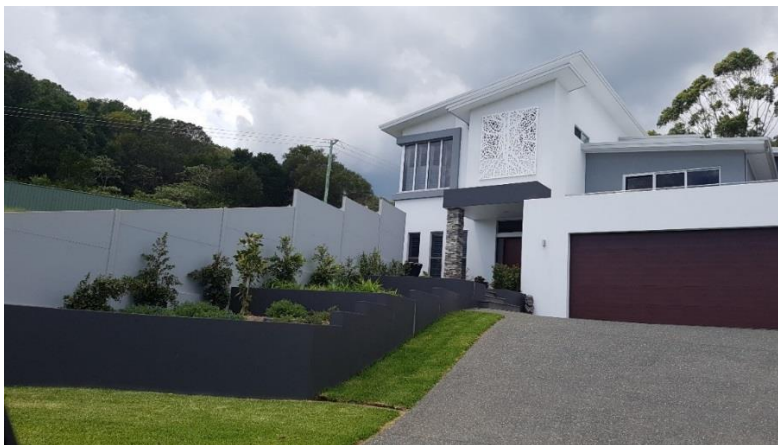
Figure 8-10 Example of a terraced biofiltration system for an individual residential lot (source: MidCoast Council)
