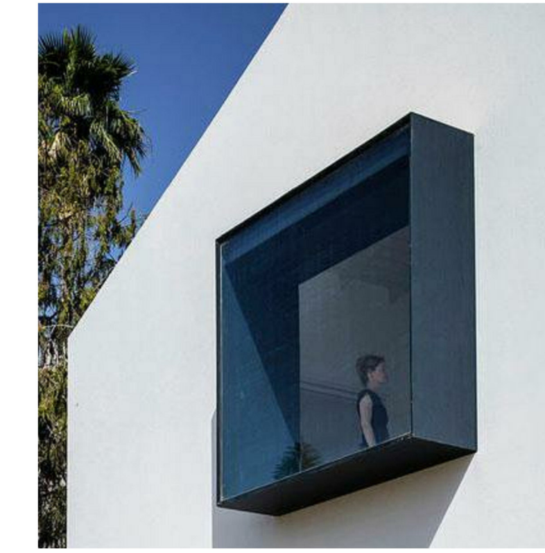
FIXED GLAZING WITH METAL REVEAL
