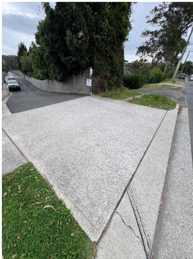
Figure 2 – Crack is evident to the layback.
