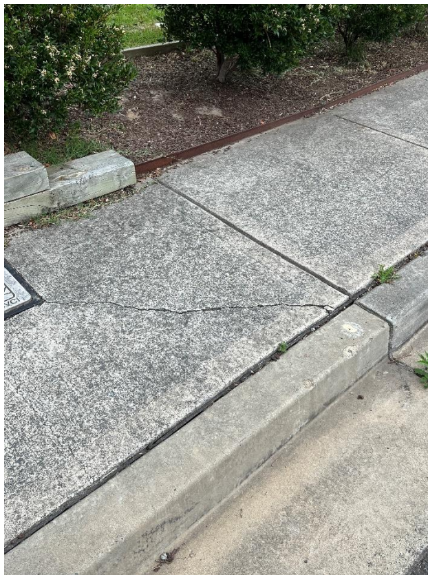
Figure 62 – Crack is evident to the footpath.
