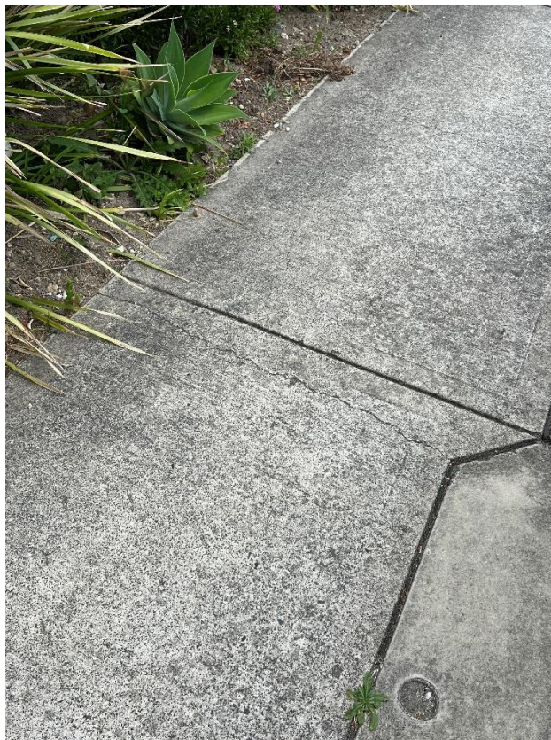
Figure 34 – Crack is evident to the footpath.
