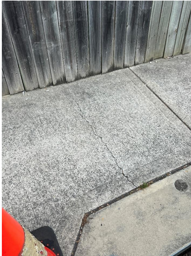
Figure 33 – Crack is evident to the footpath.
