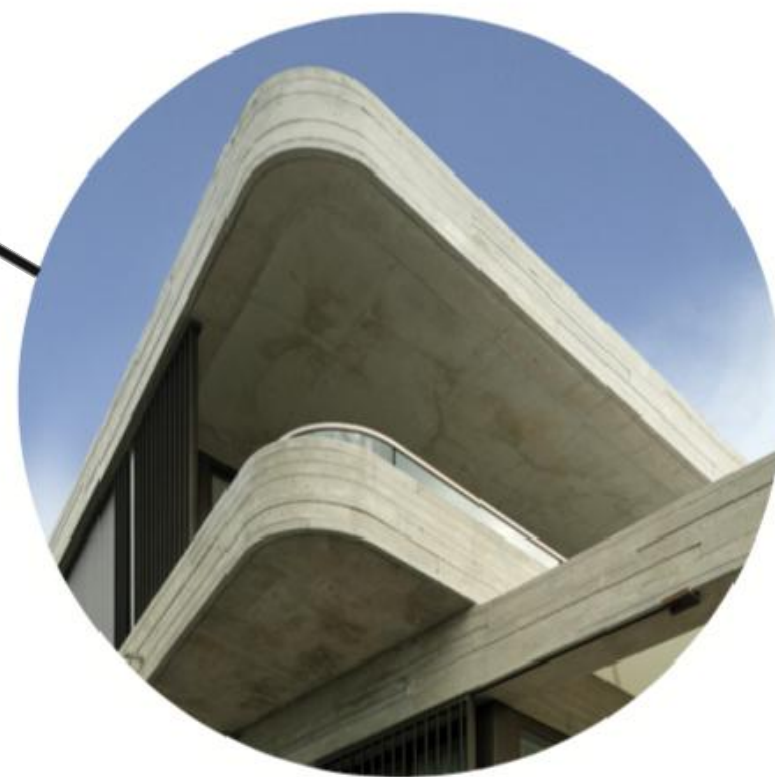
OFF FORM CONCRETE
