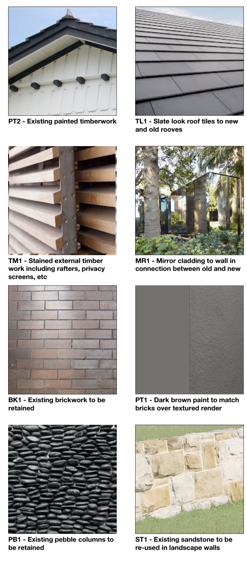
PT2 - Existing painted timberwork TL1 - Slate look roof tiles to new and old rooves TM1 - Stained external timber work including rafters, privacy screens, etc MR1 - Mirror cladding to wall in connection between old and new BK1 - Existing brickwork to be retained PT1 - Dark brown paint to match bricks over textured render PB1 - Existing pebble columns to be retained ST1 - Existing sandstone to be re-used in landscape walls
