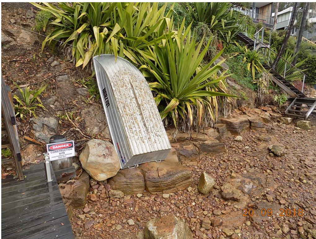
Photo 10: This photo was taken prior to the construction works to show the outcropping sandstone.
