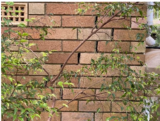
Photograph: 3 Showing crack at south-west corner1
