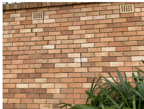
Photograph: 4 Showing stepped crack southern wall
