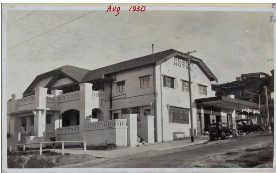
Figure 9: The western elevation of the Harbord Beach Hotel in August 1930 Source: Noel Butlin Archives
