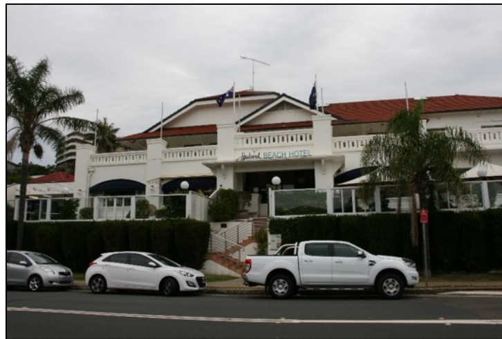
Figure 19: The front (southern) elevation of No. 29 Moore Road, Freshwater.
