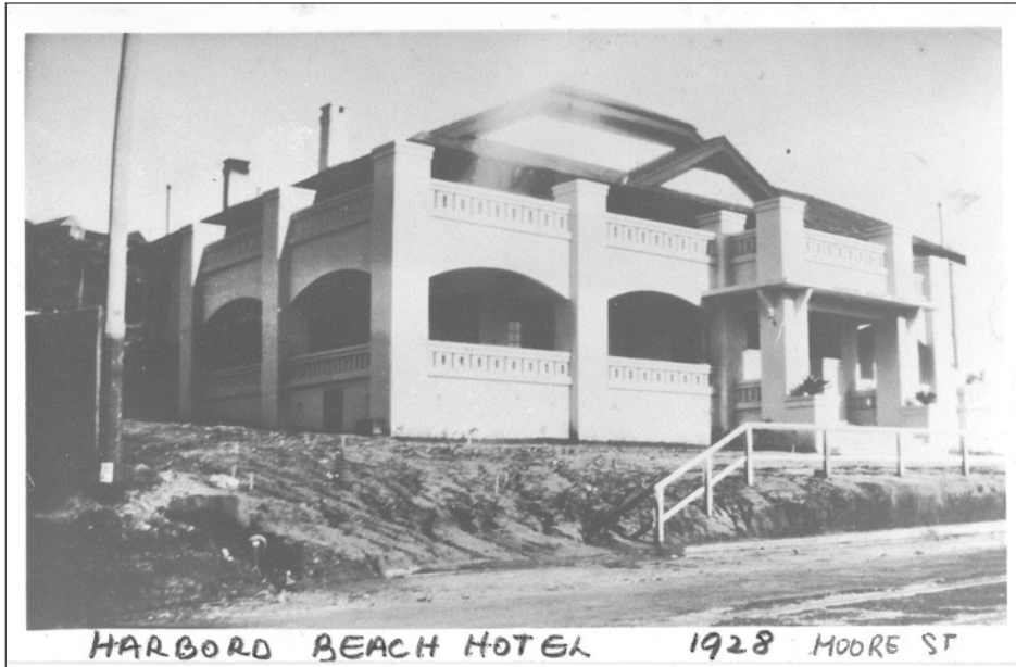
Figure 8: Harbord Beach Hotel soon after completion in 1928. Source: Northern Beaches Council Library
