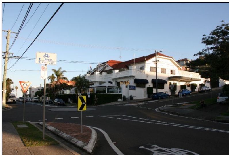
Figure 28 View of the building from the west.
