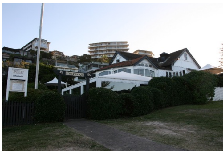
Figure 32: No. 80 Undercliff Road, Freshwater.
