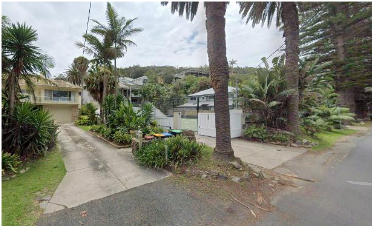
Figure 3: Subject property as viewed from Allen Avenue (south-east)
