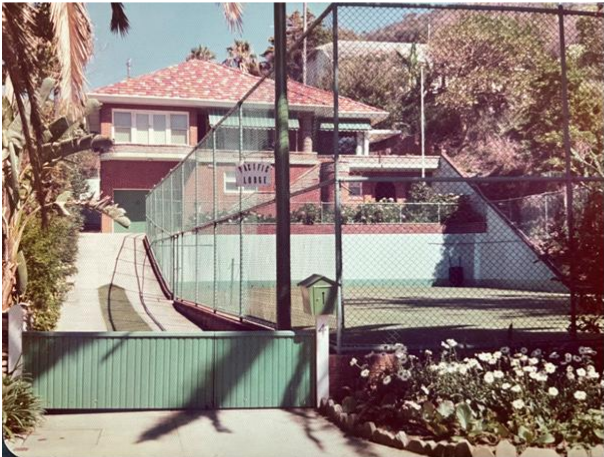
Figure 6: Photograph of completed dwelling house showing ramped driveway along the southern boundary of the property and the significant retaining wall which extended along the northern boundary before returning along the western and southern boundaries of the property to create a generally level building footprint
