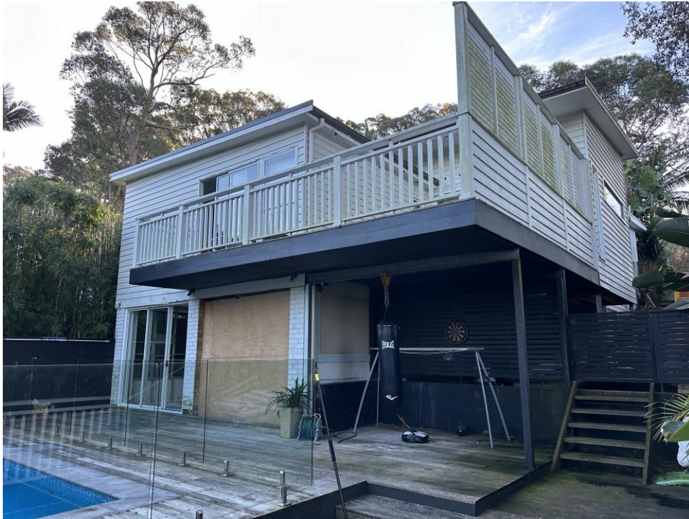
Figure 8: The rear of the dwelling, looking north-west.
