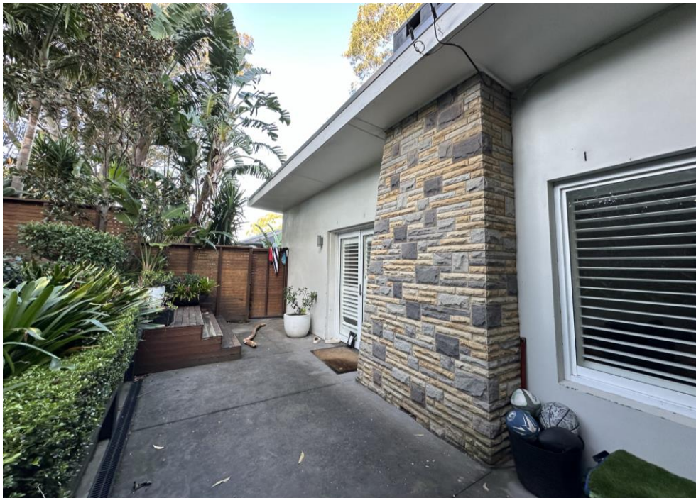
Figure 5: The dwelling façade, looking east.
