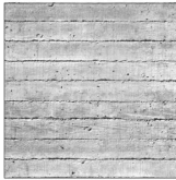
CO-01 RIBBED CONCRETE
