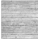
CO-01 RIBBED CONCRETE
