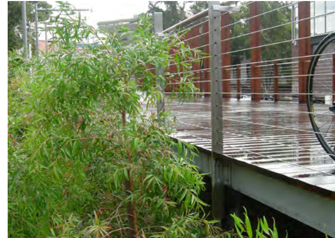
Above: WSUD bioretention swale with raised boardwalk
