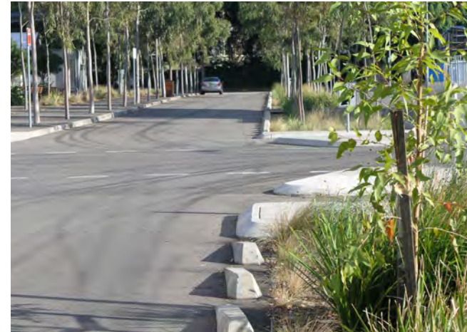
Above: Segmented kerbs to street edge allows overflow drainage into rain gardens / biofiltration
