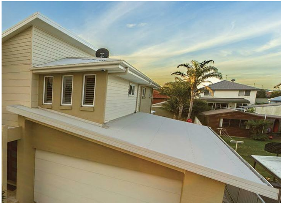
METAL DECK ROOFING - SURFMIST AS PER EXISTING
