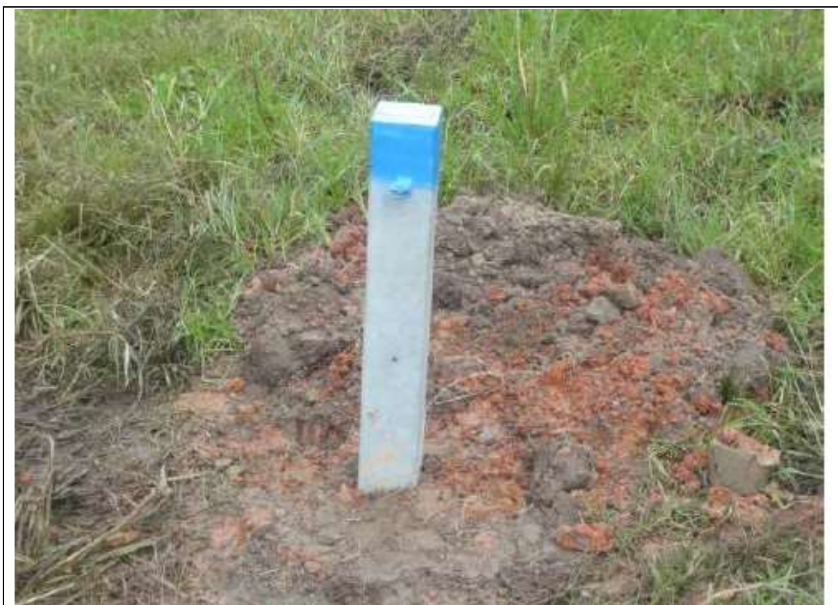
Figure 4.6 – “Monument” Style Well Pipe Cover at MW1
