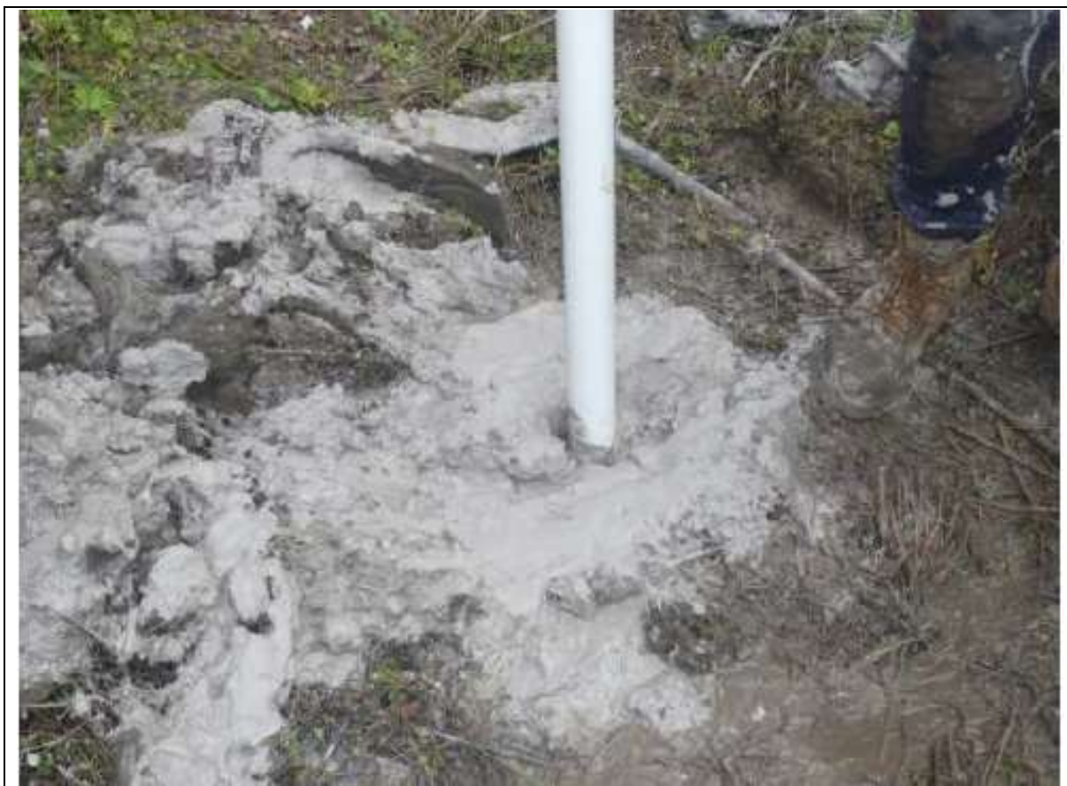
Figure 4.5 – Well Casing Pipe Installed at MW3
