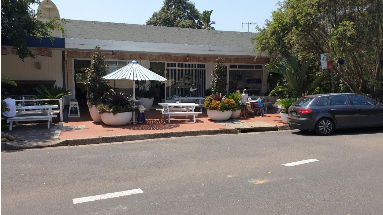
No 231 Whale Beach Rd Existing kerb inlet pit etc - 1
