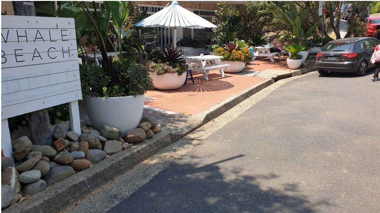
No 231 Whale Beach Rd Existing kerb inlet pit etc - 2
