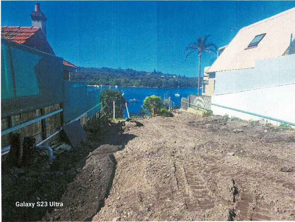
Photograph 9: Existing dwelling demolished cleared site
