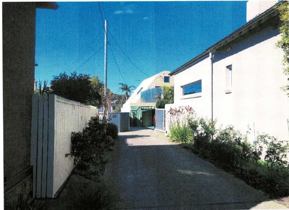
Photograph 8: Right of carriageway
