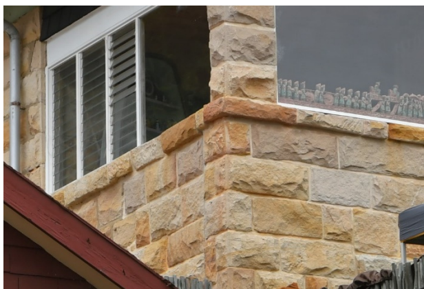
Irregular sandstone walls
